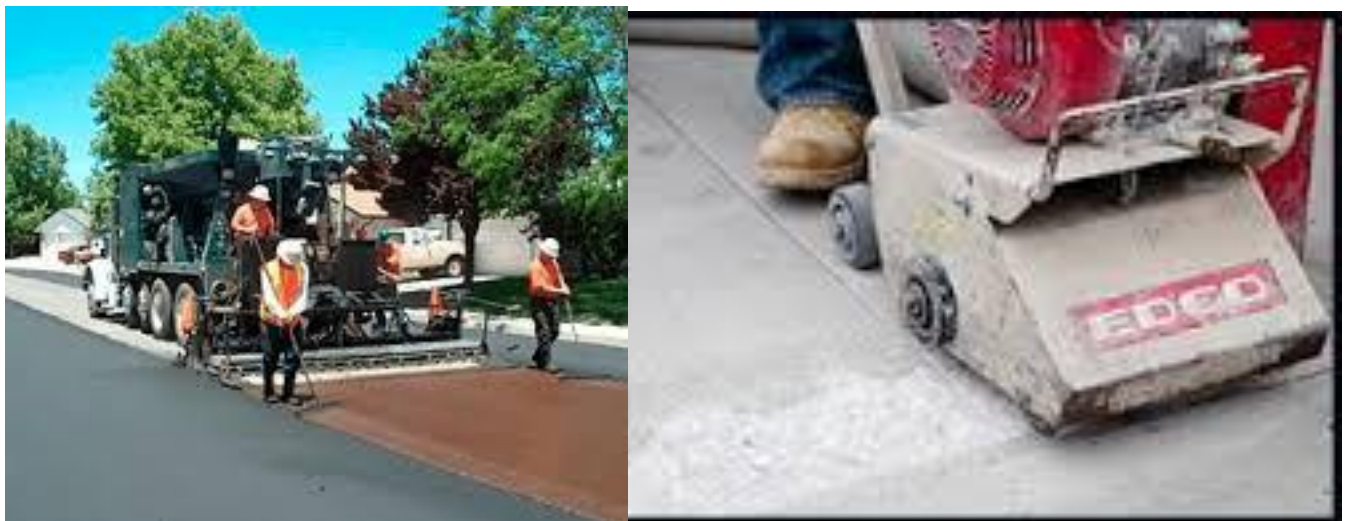
Figure 20 – Diamond Grinding and Thin-Bituminous-Surface
