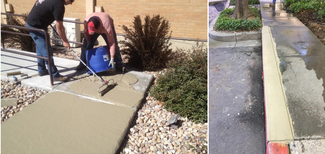
Figure 19 – Bonded Overlay
