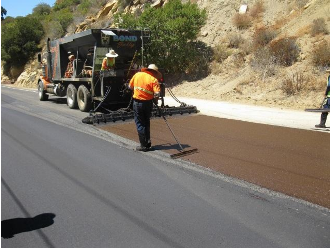
Figure 17 – Micro-Surfacing
