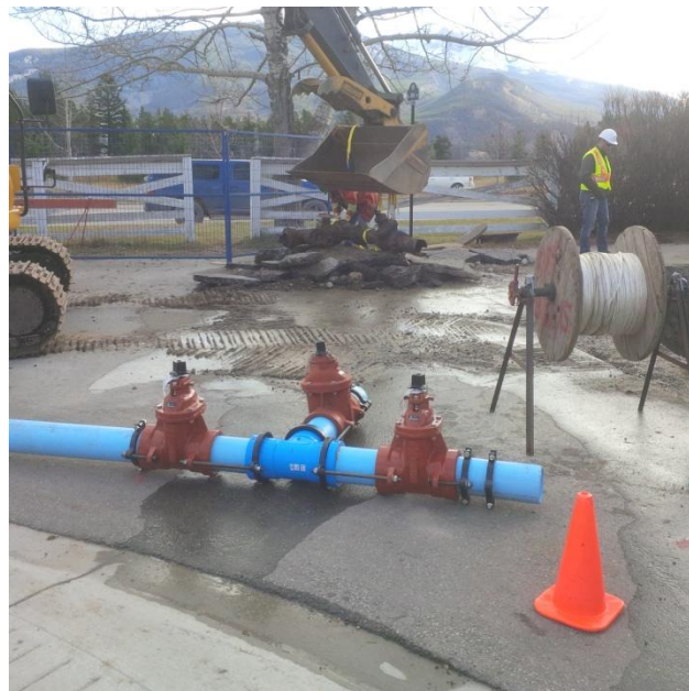
Figure 15 – Patricia Circle Water Main Pipe #2871 Valve Assembly Replacement (Year 2016)
