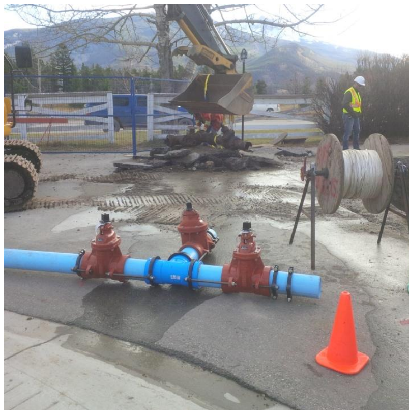
Figure 30– Patricia Circle Water Main Pipe #2871 Valve Assembly Replacement (Year 2016)
